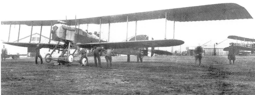
138 Above: Breguet de Chasse (Type 8) with a 225hp Sunbeam engine. Five served with 1 and 3 Wings at St. Pol, another ten with 5 Wing at Dunkirk in spring 1916 (Barry Ketley)
