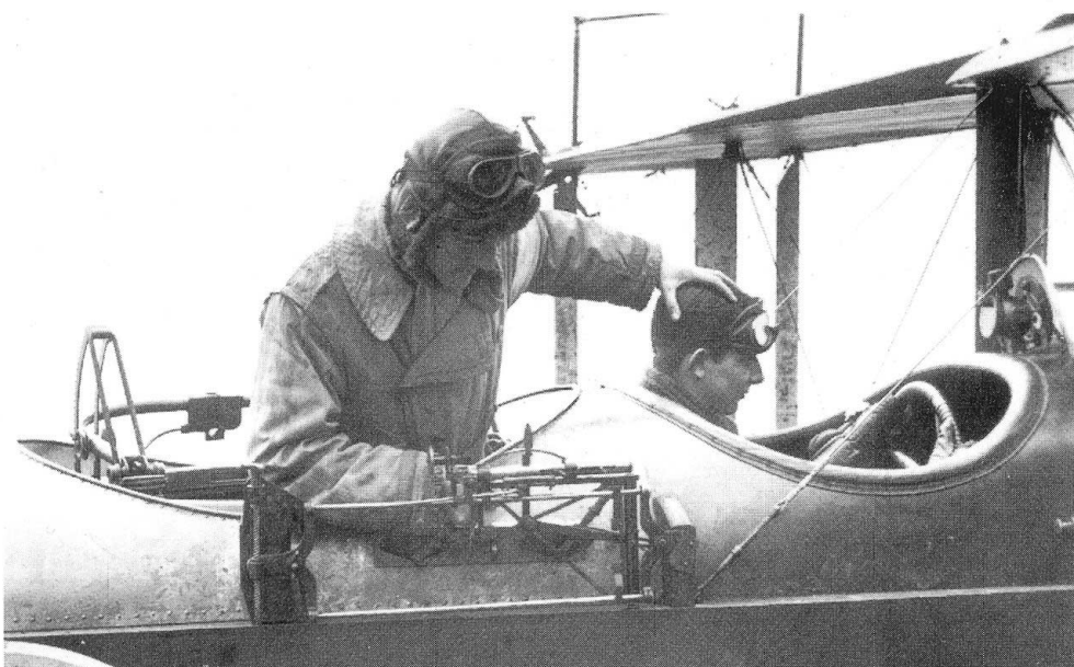
218: It was soon realised that accurate bomb dropping required a little more attention to detail than a deft lob over the side of the aircraft. Lt. Dangerfield demonstrates how the pilot of a bomber could be directed in the air. The CFS Bomb-Sight seen here was designed by 2nd Lt. G. Dobson and Lt. Bourdillon of the Central Flying School (hence its name). It was in use with a few minor improvements until the end of 1916. The sole major failing of the D.H.4, however, namely the distance between the two cockpits, meant that a different technique was necessary (IWM Q 60869)
