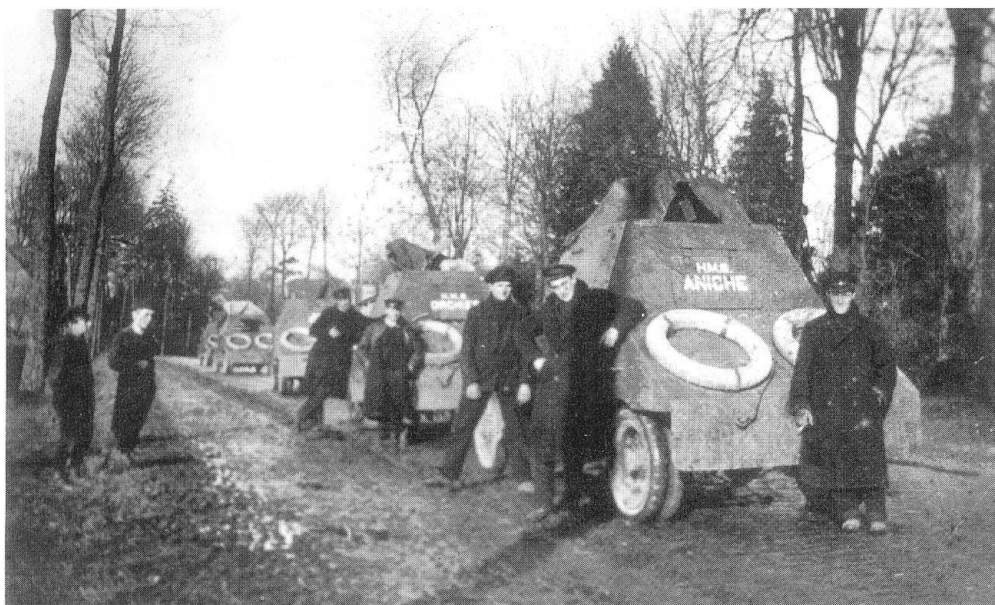
30: Admiralty pattern Talbot armoured cars on the road. HMS Aniche and HMS Orchies in the background (both named after towns in their area of operations) and the others seen here were of the second type sent out to France. Samson did not like the lack of driver protection and had six built up in the Dunkirk shipyards to the standard seen here. The white objects on the hull plate are spare tyres, not life-belts. Samson Collection (IWM HU)
