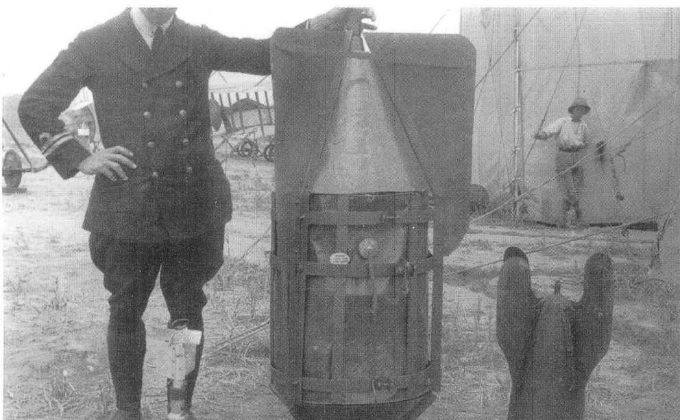
54: A home made incendiary bomb constructed from a 10lb bomb and a petrol tank. The pilot was warned to head straight out to sea in case of accidents. On impact it failed to go off immediately and Turkish troops took it in turns to have their photograph taken while standing on it. Sadly, one such group eventually did set it off (IWM Q 44277)
